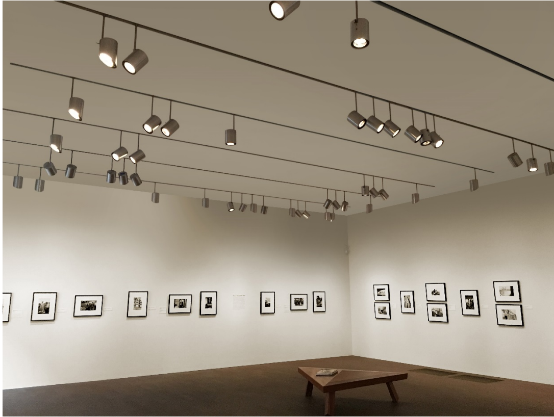
Conventional gimbaled spotlights Entire fixture pivots to point beam
